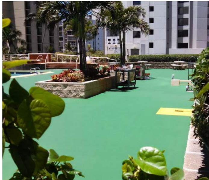
Almost pau: concrete repaired and painted
